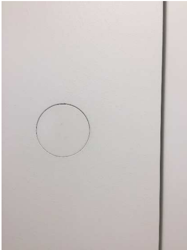
Disc installed flush
